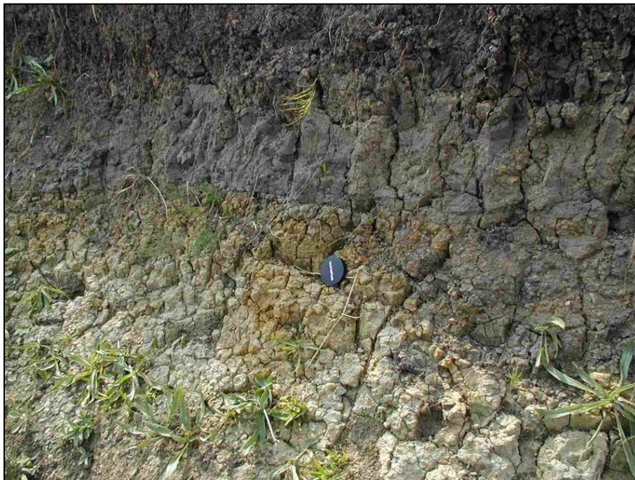
Figure 2: Soil cracking due to desiccation (Camera lens cap is 5.5 cm in diameter).
