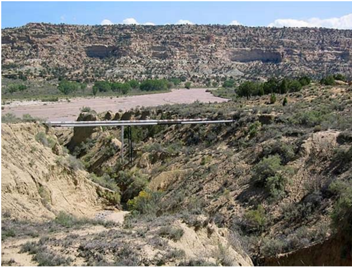
Figure 4. This New Mexico pipeline crosses the channel near the elevation of the highest terrace, which places it above even the most extreme flood events.
